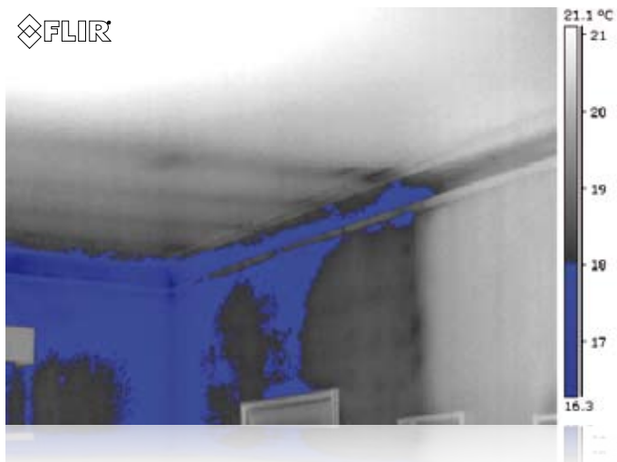
The image shows reflections on an inner wall (to the right) from the window to the left.
