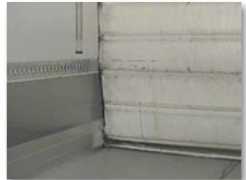
◆ Airleak in insulation curtain separating two temp zones in refrigeration box
