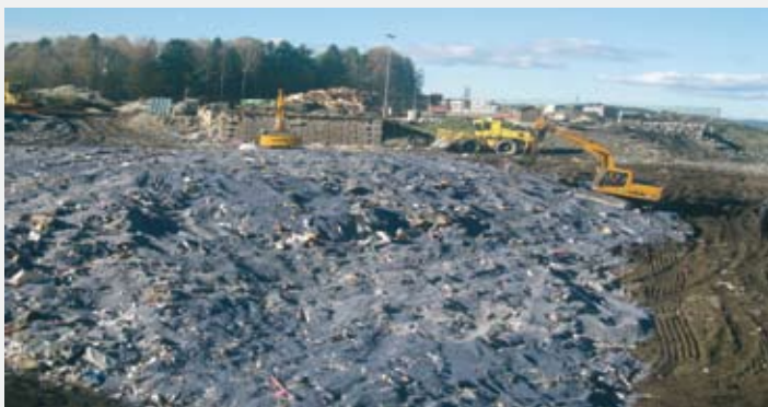
Covering and sealing a landfill site with clay
