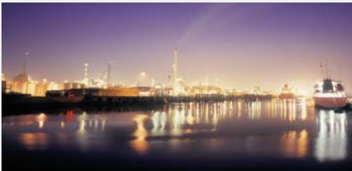
A modern complex petrochemical facility
